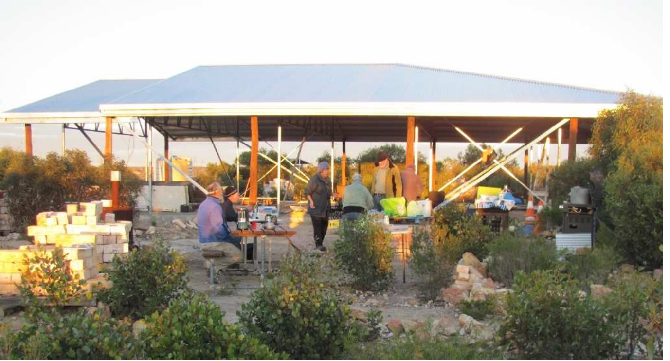
Early morning light on the recently roofed building.
