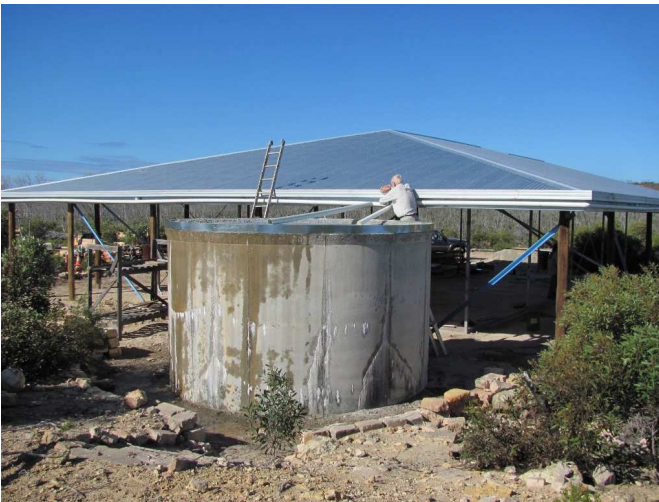
Tanks are attached to the new roof.
